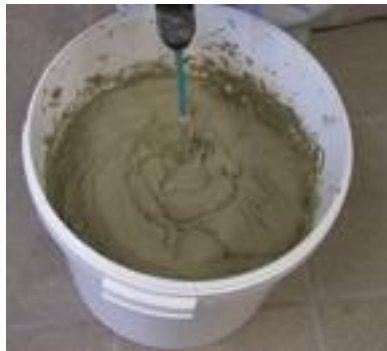
Mix the mortar with an agitator. Put comp. A + B into a 30l pail and mix thoroughly for 2 minutes- done.
